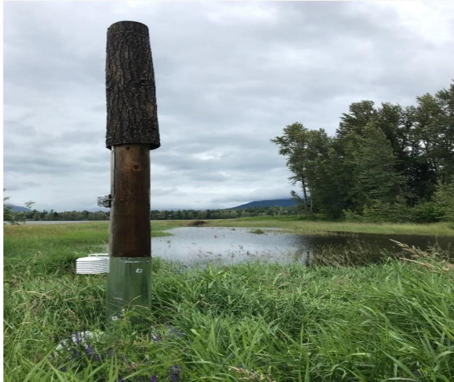
Photo 1 BrandenBark™ Artificial Bark Pole Installed at Montana 3 (M3-Bark1)
